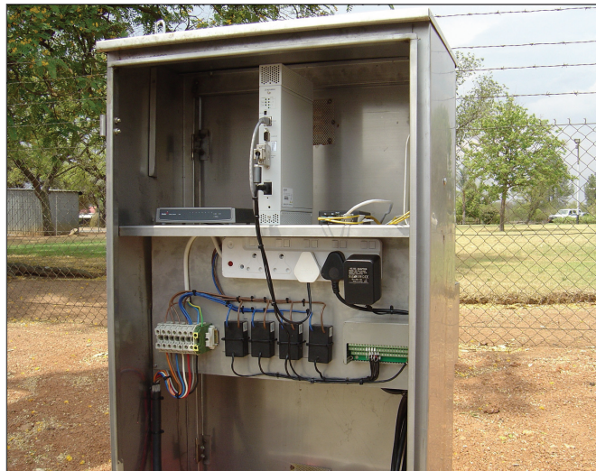
The pilot installation at Rooiwal. The signals is fed to the street box by fibre link and inserted on the the distribution network
